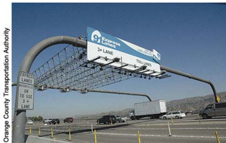
Image 2 SR 91 Toll facilities, Orange County, California
